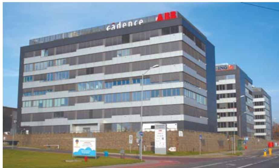
GPP Business Park, budynek Alder
